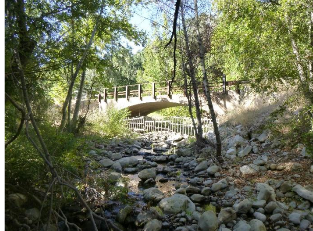
Figure 2. View, facing upstream, of the reconstructed channel and the upgraded bottomless arch culvert. Post-treatment photo date: 9/26/2023
