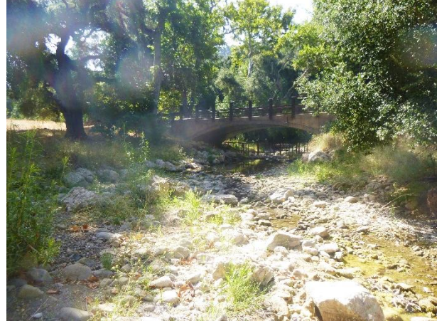
Figure 2. View, facing upstream, of the reconstructed channel and the upgraded bottomless arch culvert. Post-treatment photo date: 9/25/2023
