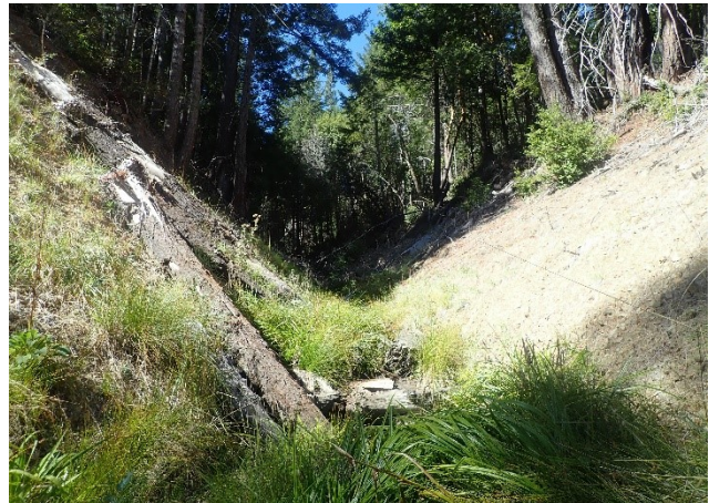
Figure 2. A restored stream bed with a 2:1 bank ratio. Placed woody material is visible along with returning vegetation. Post-treatment photo date: 09/30/24.
