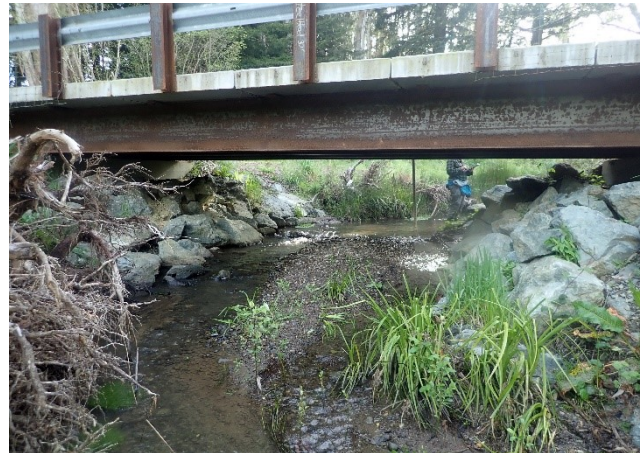
Figure 2. New 30' spanning bridge that opens fish passage above crossing. Post-treatment photo date 4/16/2024
