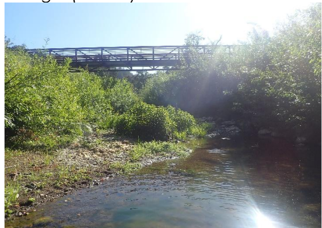
Figure 2. Reconstructed channel after dam removal with new spanning pedestrian bridge.
