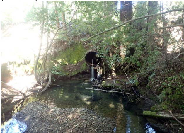
Figure 1. Outlet of perched culvert prior to removal. Pre-treatment photo date: 02/26/2020.
