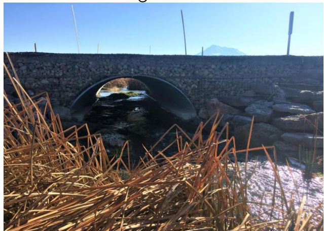
Figure 2. Post-construction view of 10' X 36" multi-plate arch culvert outlet. Post-treatment photo date: 2020
