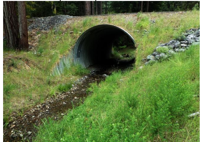
Figure 2. Culvert installed to allow for fish passage. Post-Treatment photo date: 05/30/2023
