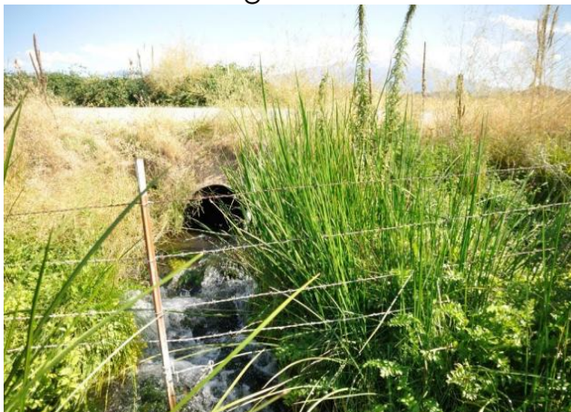
Figure 1. Pre-construction view of 30" CMP culvert outlet. Pre-treatment photo date: 2014
