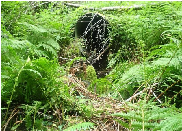
Figure 1. Perched culvert prior to decommissioning on logging road 4200. Pre-treatment photo date: 06/15/2020
