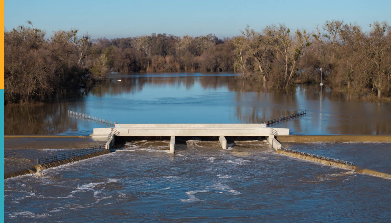
Sacramento River overtops the Fremont Weir and inundates the Yolo Bypass floodplain through the Big Notch Project; Credit: DWR.
