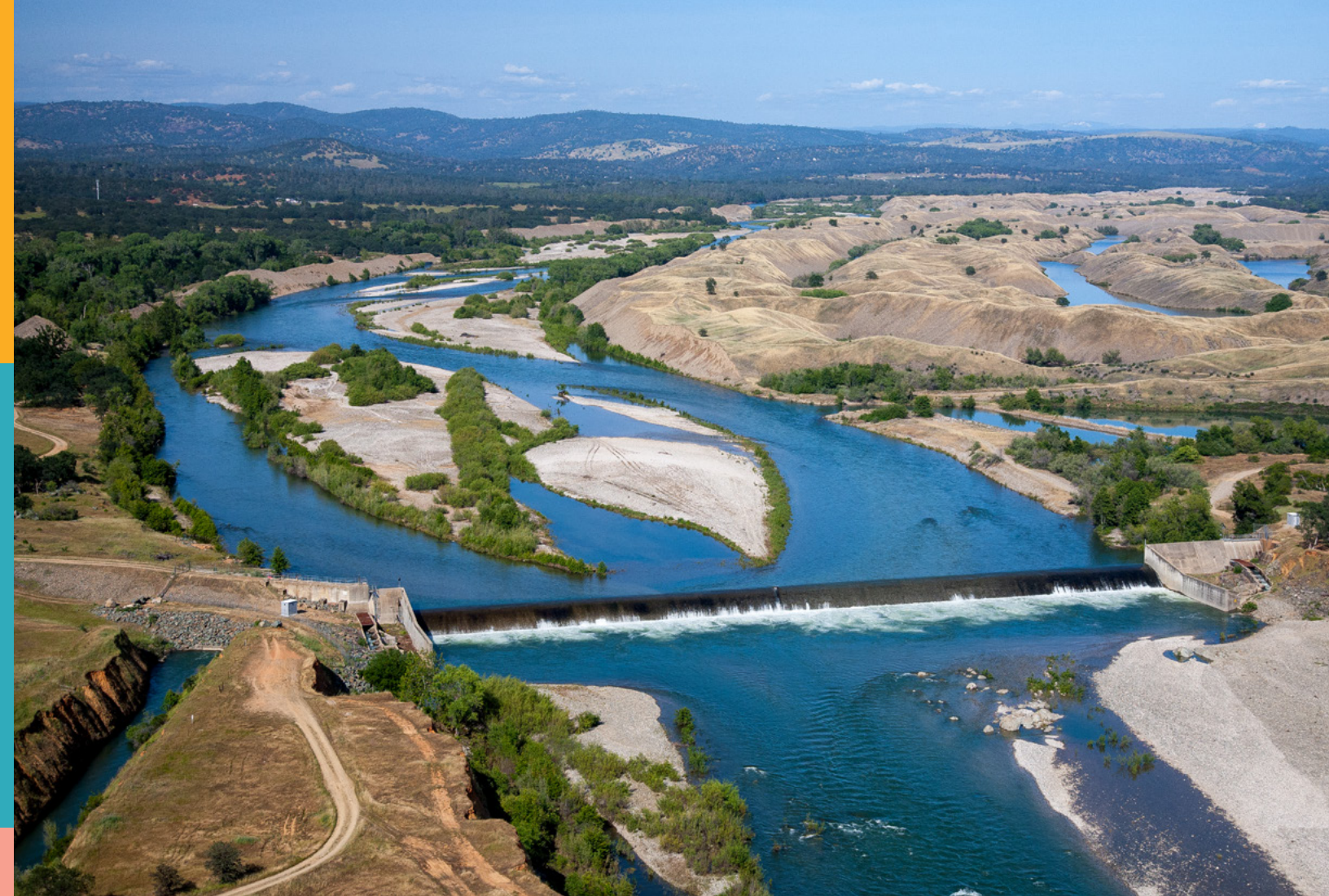
Daguerre Point Dam slated for fish passage improvements under the Yuba River Resilience Initiative, with construction anticipated to begin fall 2026; Credit: DWR.
