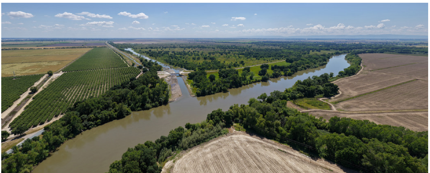
Sacramento River inundation through the Yolo Bypass Salmonid Habitat Restoration and Fish Passage Facility at Fremont Weir; Credit: DWR.
