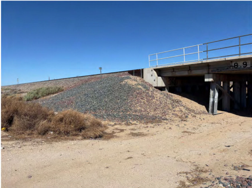
TYPICAL RAILROAD EMBANKMENT BARRIER
