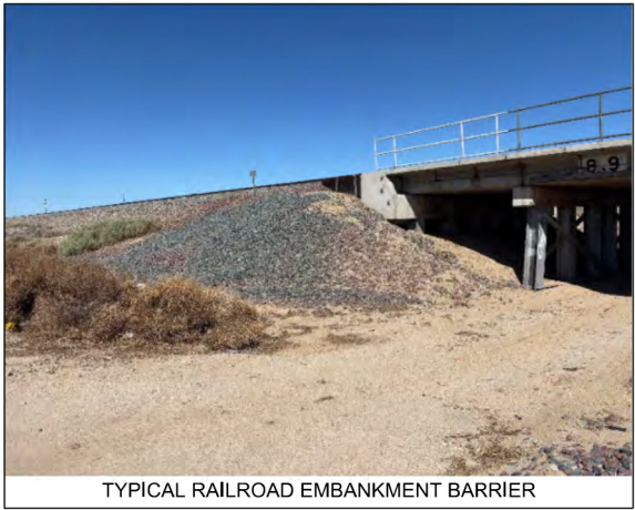
TYPICAL RAILROAD EMBANKMENT BARRIER
