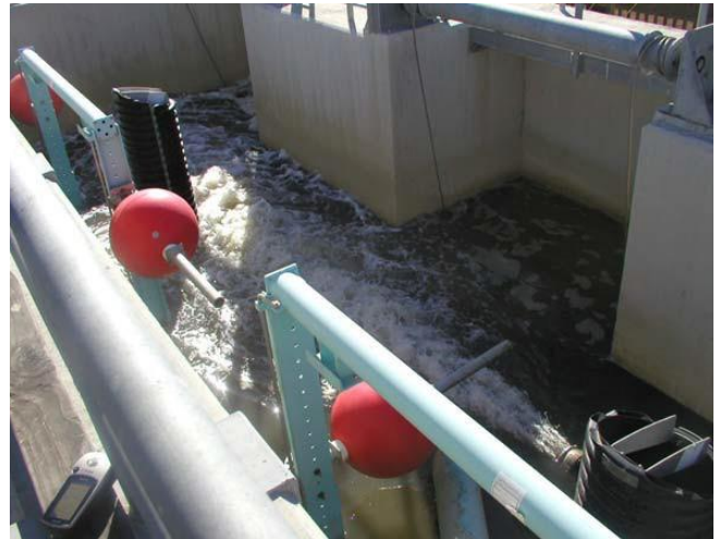
Operating tide gate
