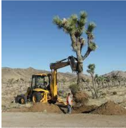
Figure 6: Salvage tree being removed from the ground by an excavator (Photo credit: National Park Service)
