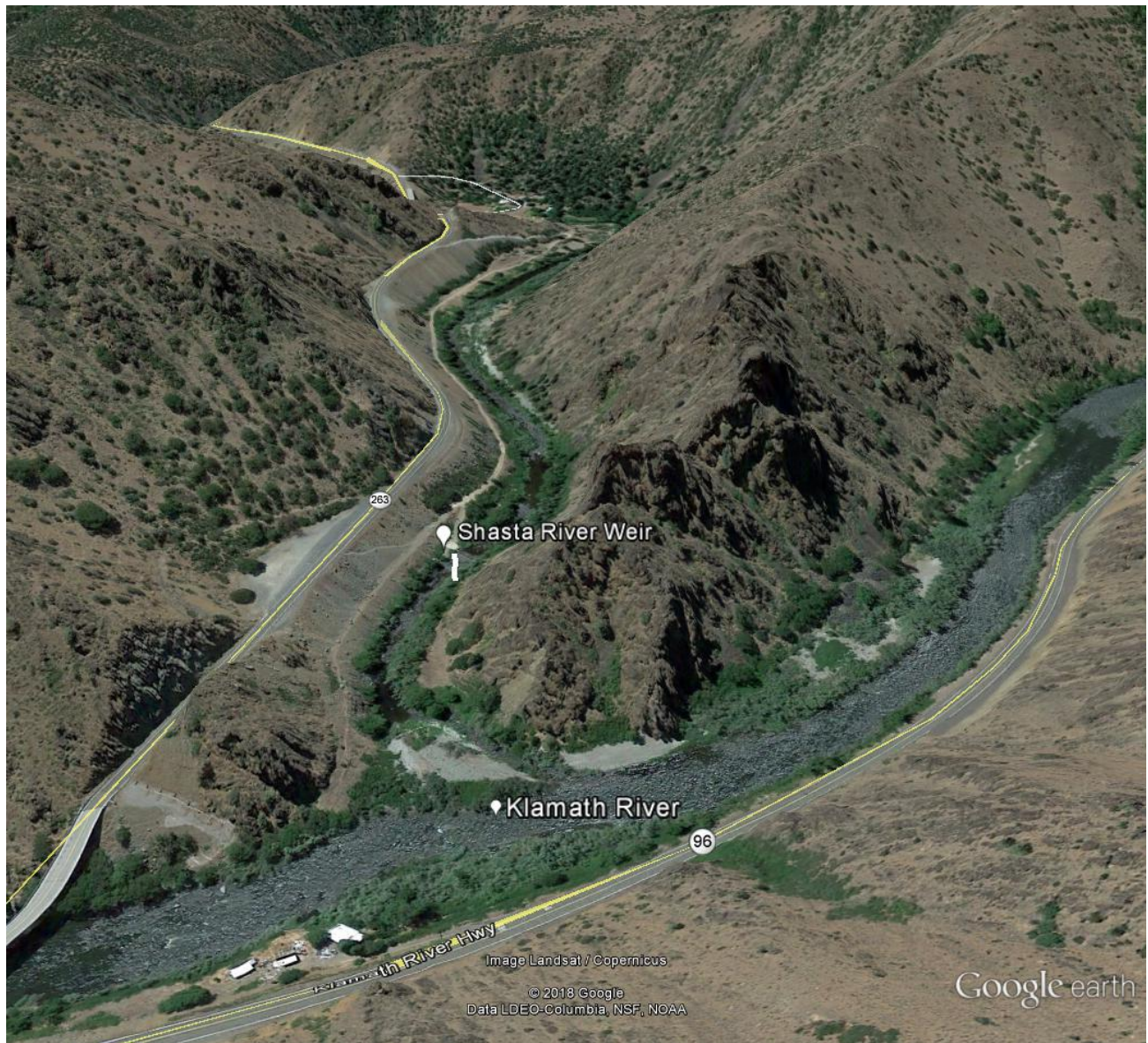
Figure 2. Google Earth Image Looking South at the Shasta and Klamath Confluence.
