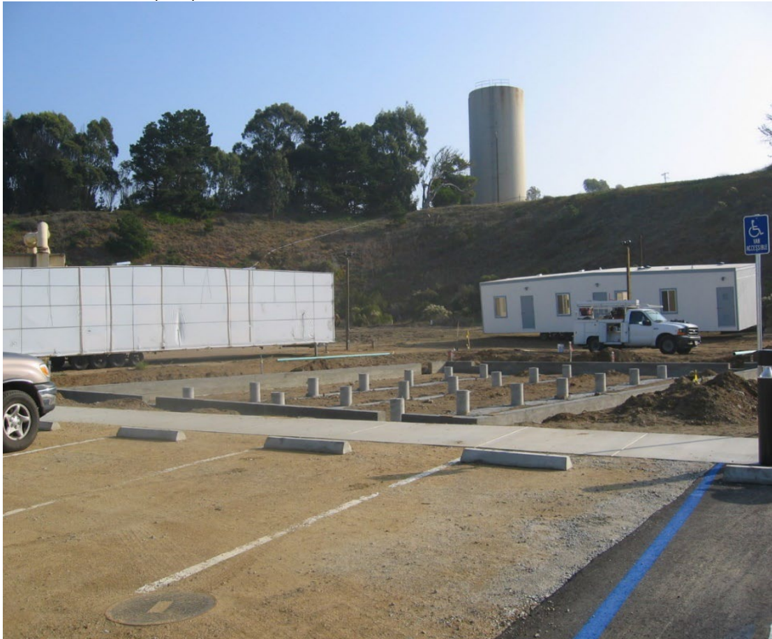
Photo 36. Site preparation with the modular trailer installed at PWC.
