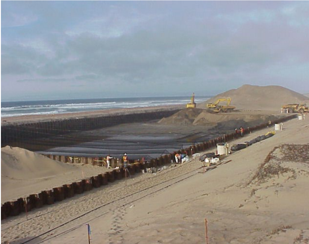
Photo 5. 5X East plume excavation.
