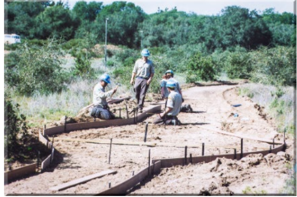
Photo 42. Pathways installed with help from California Conservation Corps.
