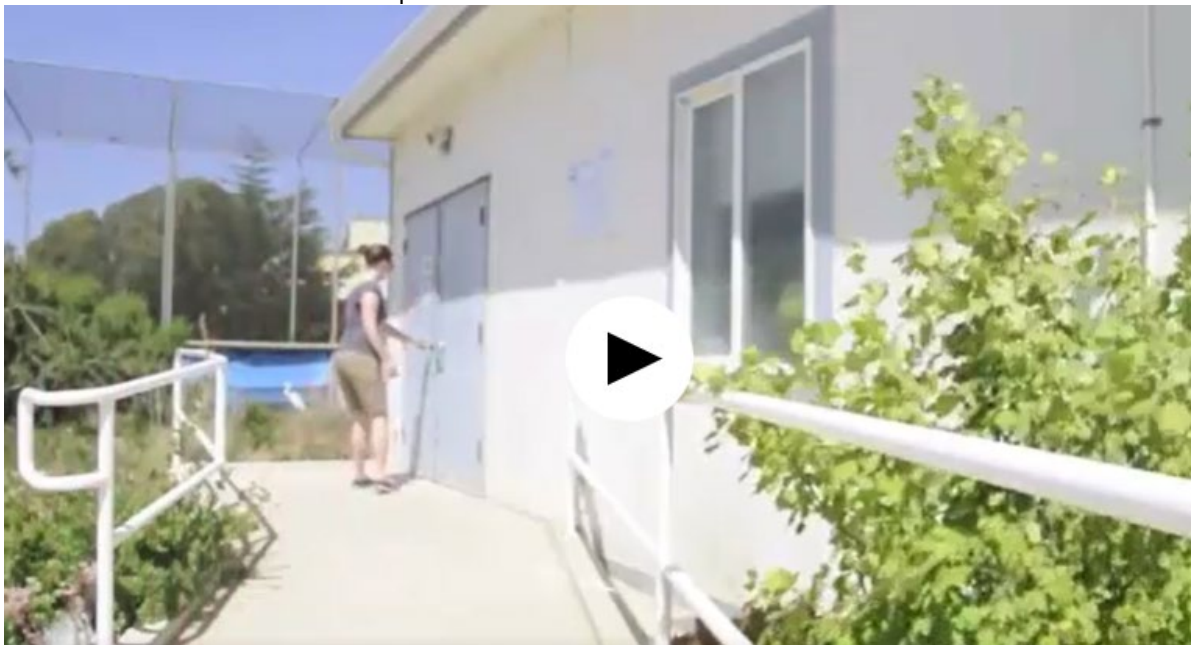
Photo 37. Outside of completed modular at PWC.
