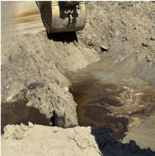
Well A excavated, with oil in the excavated sump.
