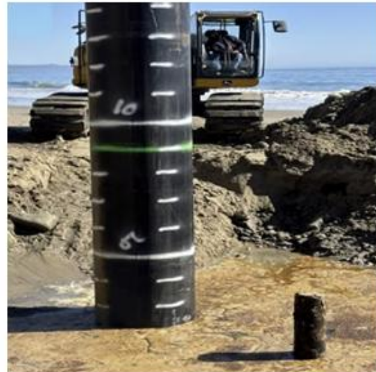
Well B wellhead being covered with 24-inch casing ready to be pile driven.
