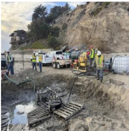
Both well caps installed and wells ready for cementing operation.
