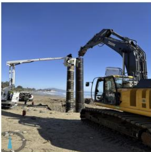
Well A 24-inch casing Installation.
