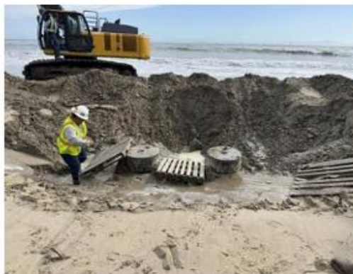
Removing refuse from the wells' location.
