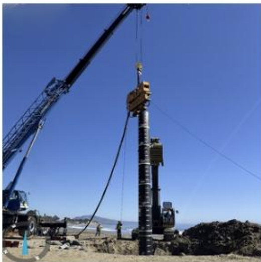
Well B 24-inch casing being pile driven to the blue clay depth.
