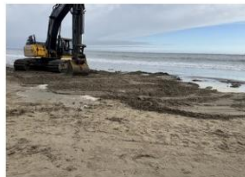
Final well location condition.
