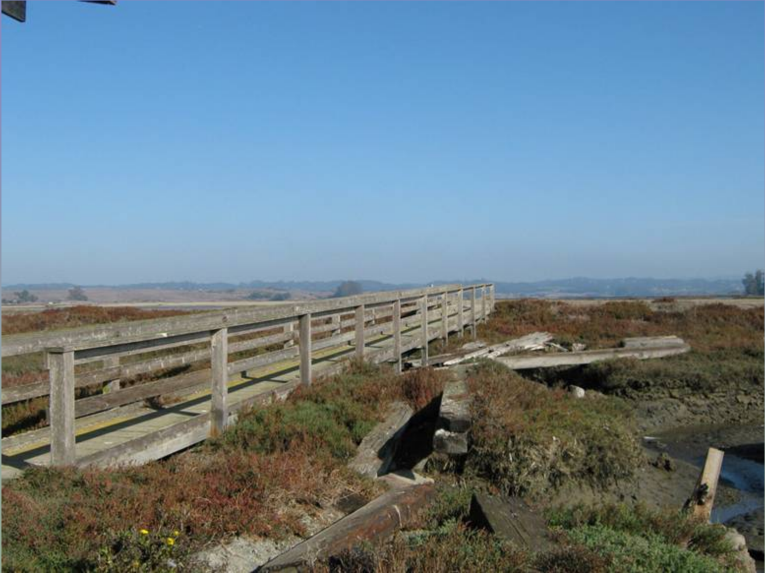
Old wooden access bridge to be replaced by new ADA compliant earthen ramp.
