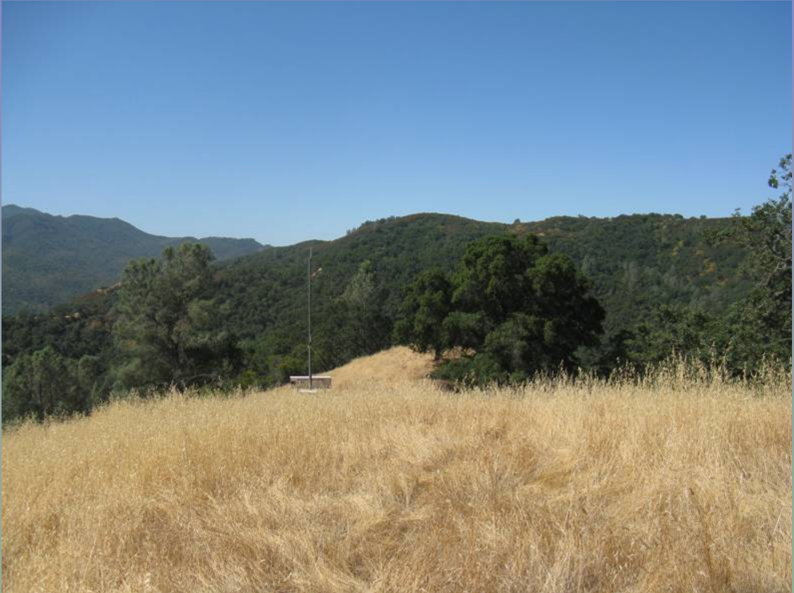
Example of Solar Powered Communications Station.
