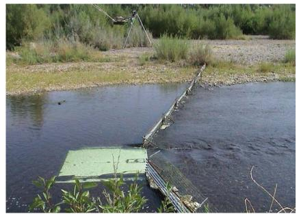
**Figure 7**. An example of a partial horizontal bar weir currently in use in the upper Sacramento River basin (Cottonwood Creek) operated to monitor fall-run Chinook salmon. The weir directs fish through the central opening where they may be filmed by overhead and underwater cameras. Photo credit: Doug Killam, CDFG.
