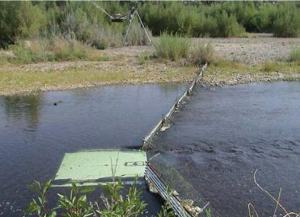
**Figure 7**. An example of a partial horizontal bar weir currently in use in the upper Sacramento River basin (Cottonwood Creek) operated to monitor fall-run Chinook salmon. The weir directs fish through the central opening where they may be filmed by overhead and underwater cameras. Photo credit: Doug Killam, CDFG.
