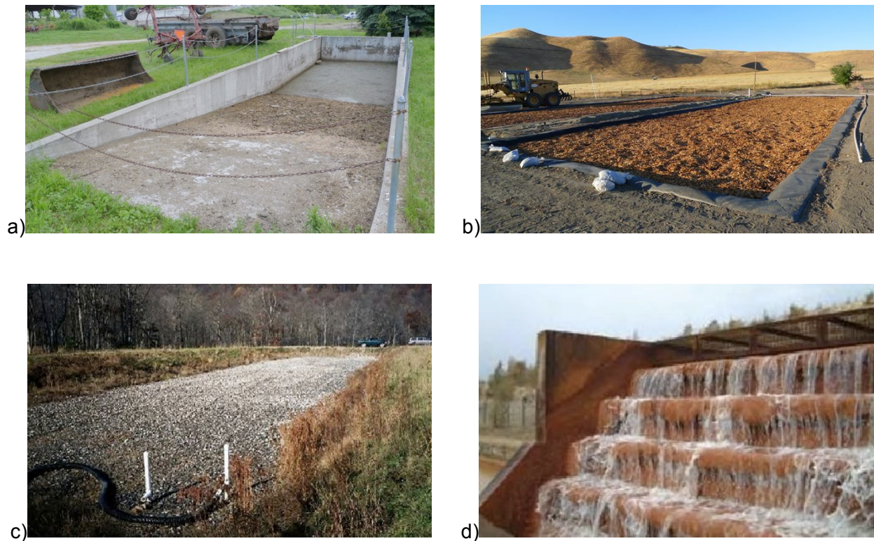
Figure C-5. Views of treatment components proposed for passive treatment of mine drainage water: (a) sedimentation basin with water level control and access ramp for removal of precipitate, (b) anoxic woodchip reactor, (c) limestone contactor, Cavanagh et al., 2010, and (d) cascade aeration, Cavanagh et al., 2010.
