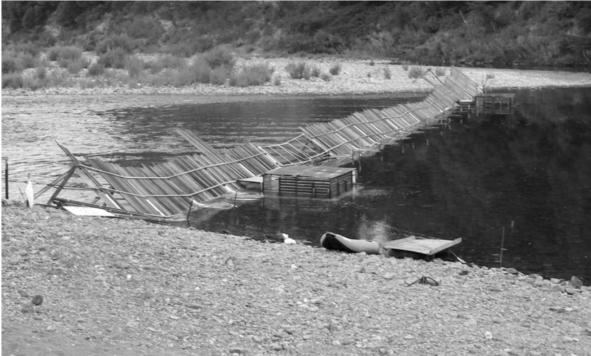
Figure 4. Photograph of Alaskan-style weir showing the trapping boxes on upstream side of the weir.
