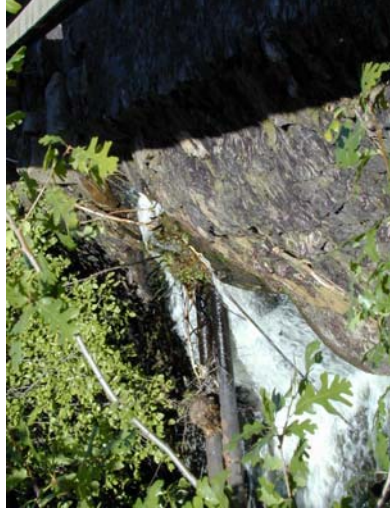
Photo 9- Cottonwood Dam-Dam is 20 feet high and appears to be a complete barrier at normal flows.
