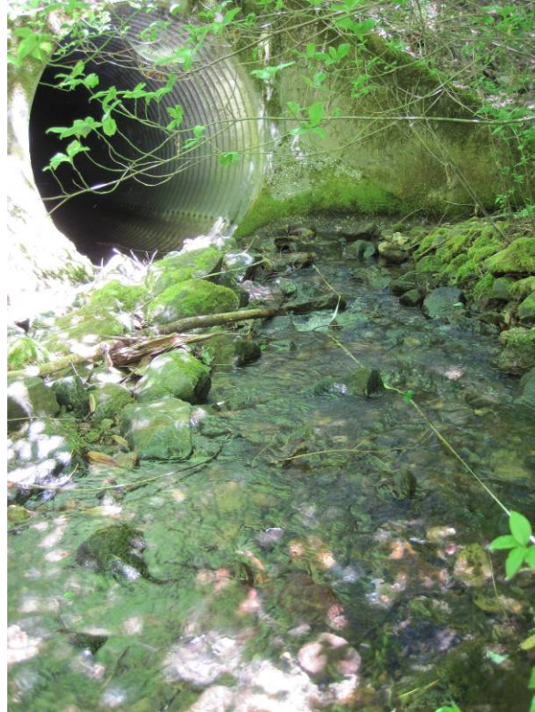
Figure 2. Culvert inlet of Indian Creek_Trib_2
