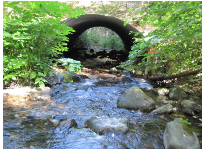
Figure 4. Culvert inlet of Indian Creek_1
