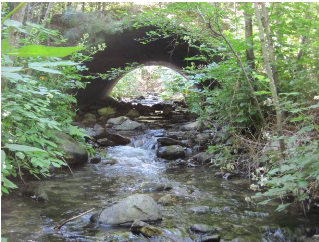
Figure 3. Culvert outlet of Indian Creek_1
