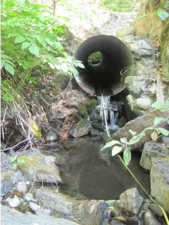
Figure 1. Culvert outlet of Blue Ravine _1
