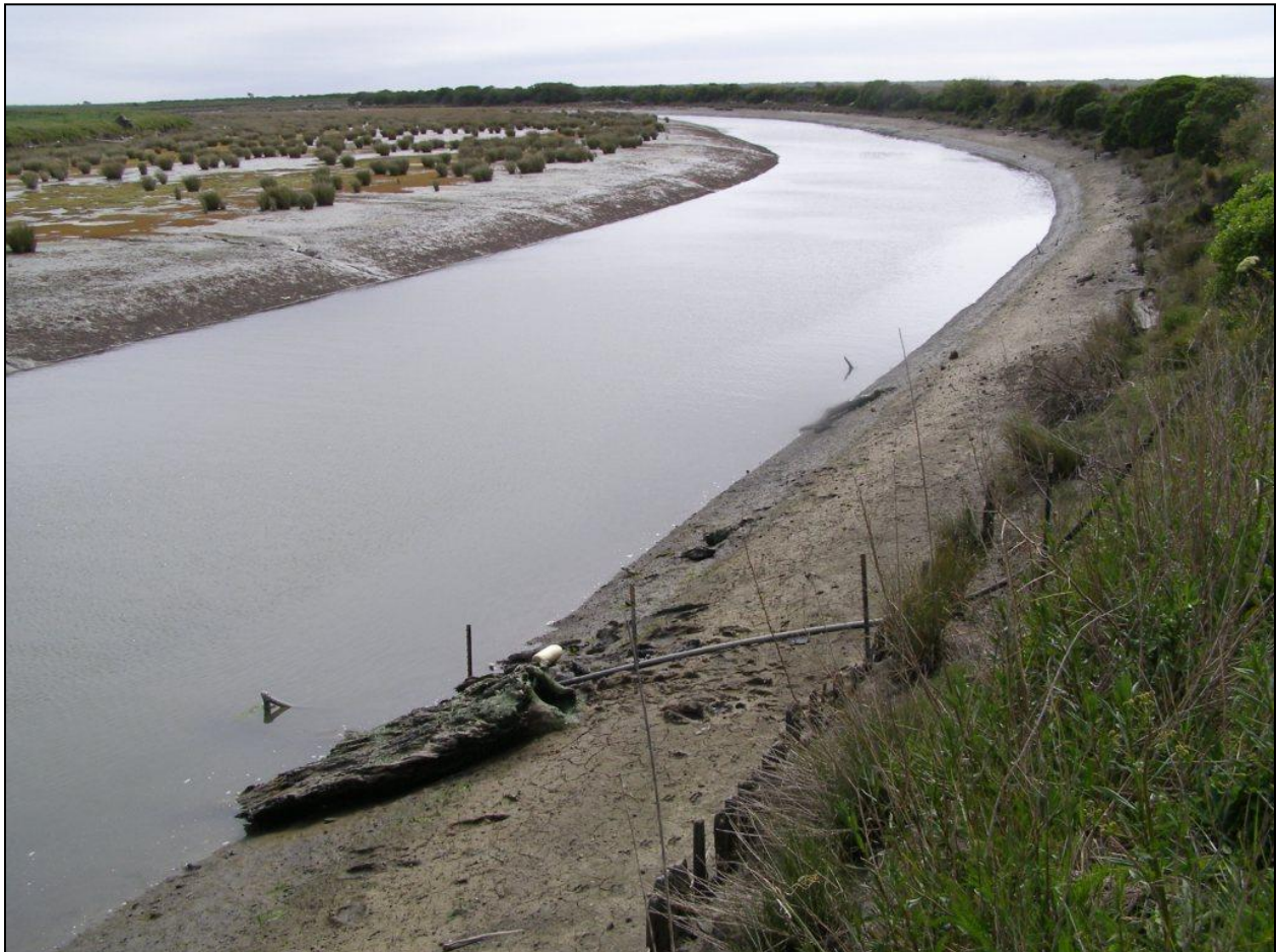
Figure 3-2. Site 1 McNulty water level station location photo. Photo date: May 13, 2008.
