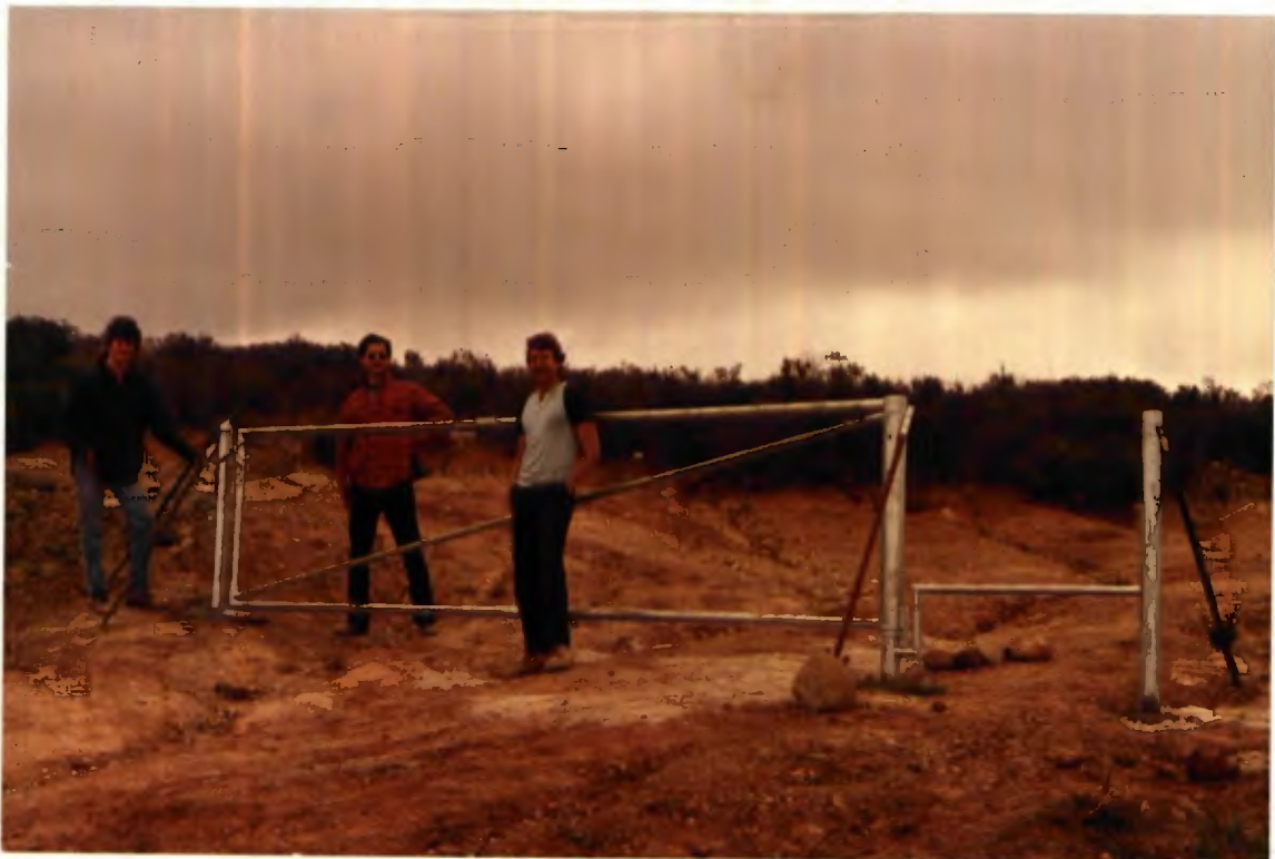
Installation of metal gates at access points of McGinty Mountain Preserve
