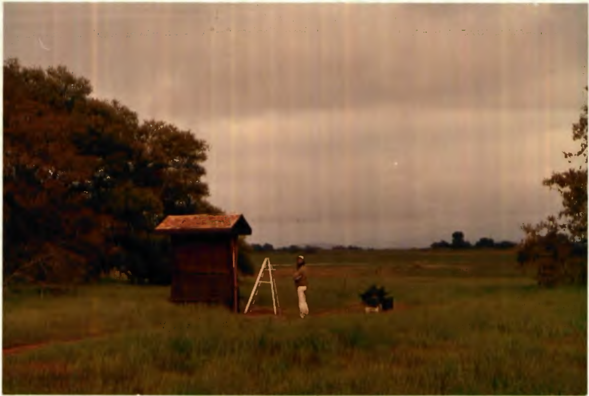
Figure 3. Carpenter John Cruzen at work on kiosk.
