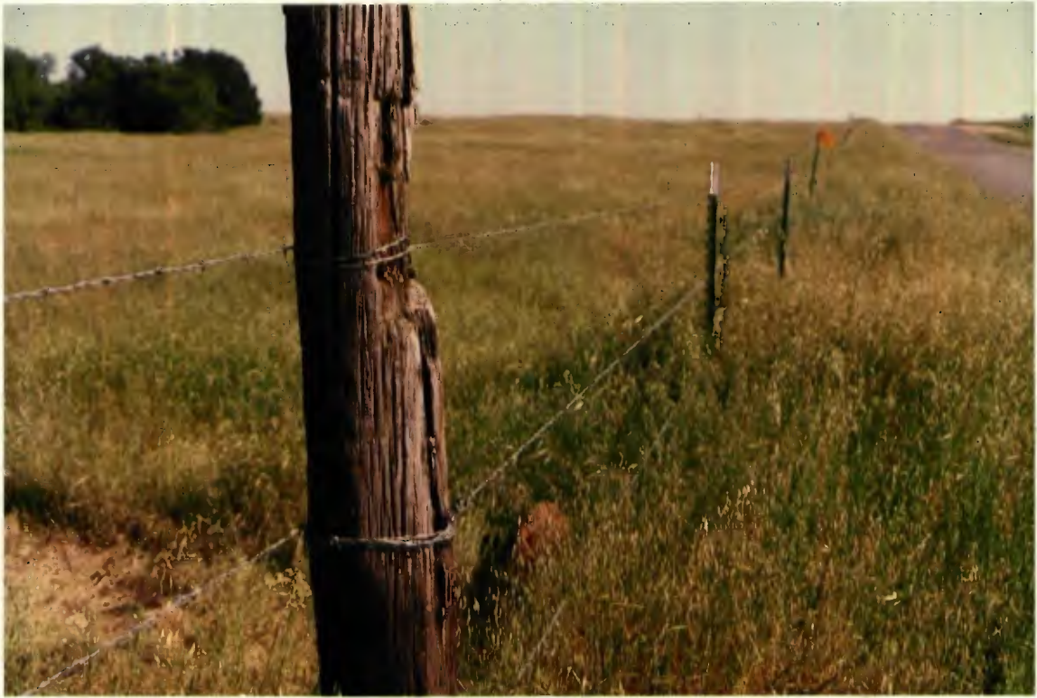
Figure 1. New fence on Mesa de Colorado.
