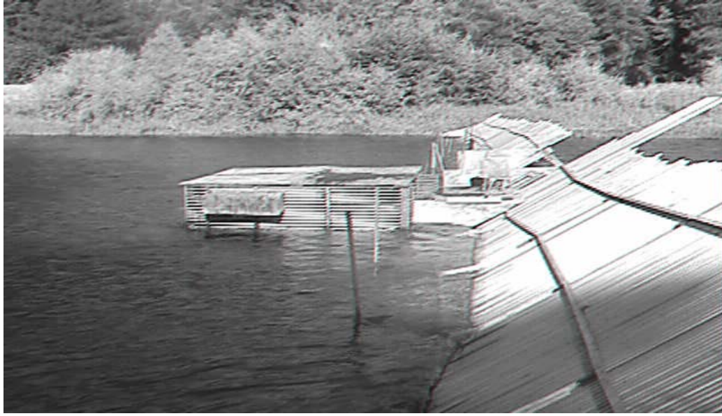
Figure 4. Photograph of Alaskan weir showing the trapping box on the upstream side of the weir.
