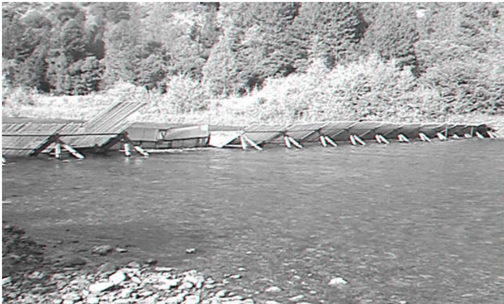
Figure 3. Photograph of upstream view of Alaskan weir. Note the panel boat gate (left center of picture).
