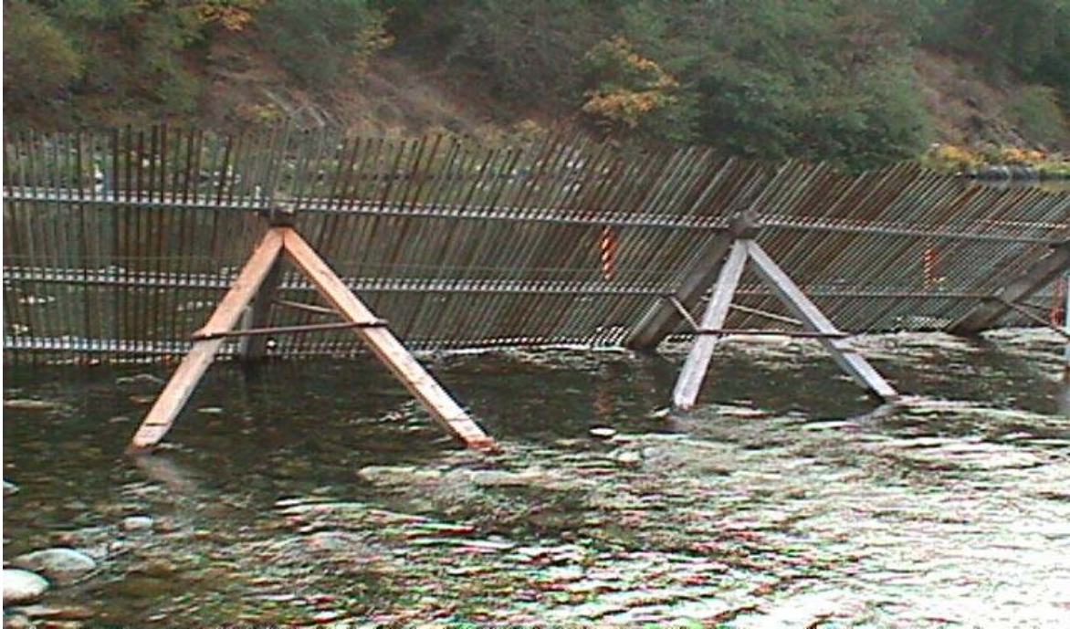
Figure 2. Photograph of Alaskan style weir tripods, support channels and conduit.
