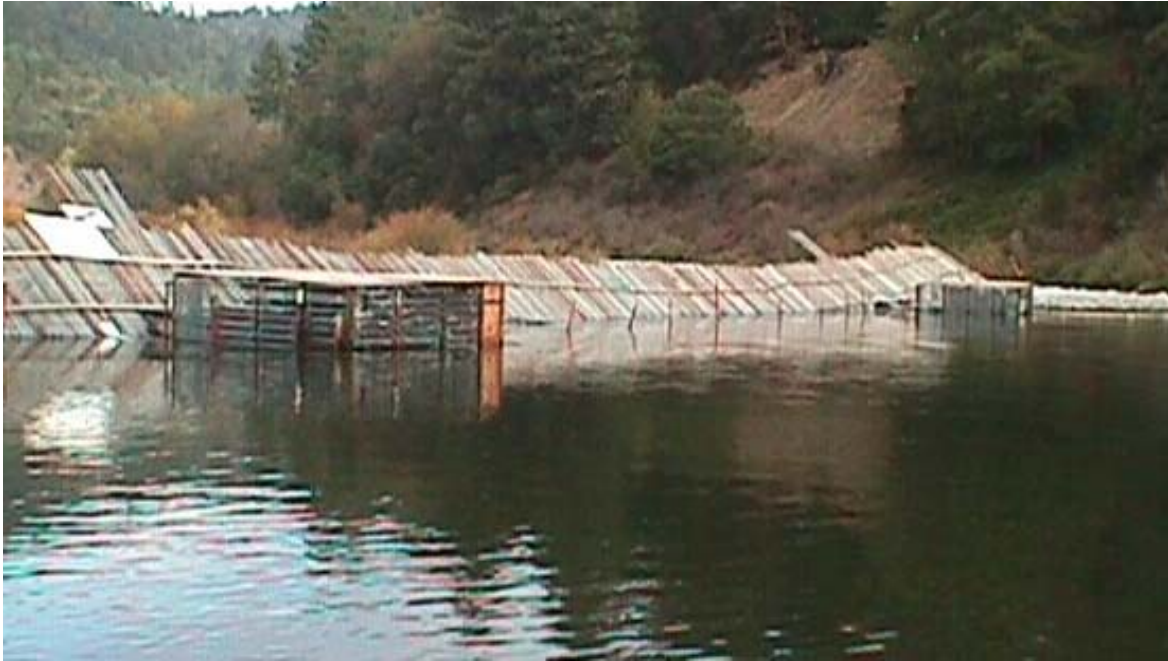
Figure 4. Photograph of Alaskan weir (taken upstream) showing the trapping boxes on the upstream side of the weir.
