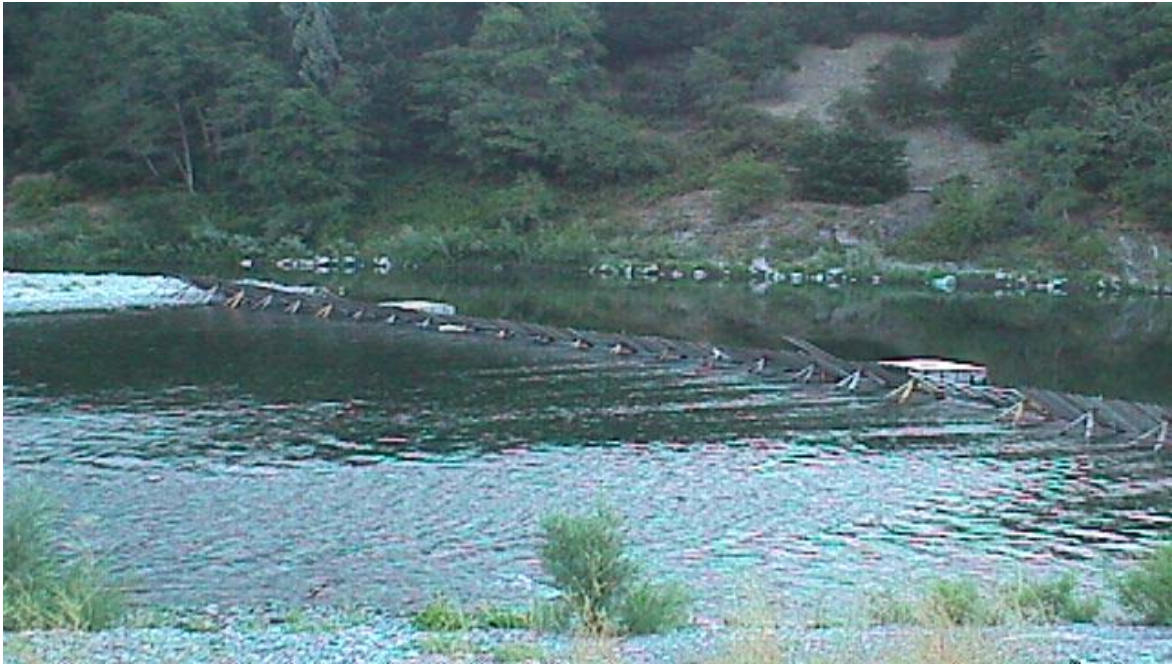
Figure 3. Photograph (taken from downstream) of Alaskan weir. Note the boat gate (right side of picture).
