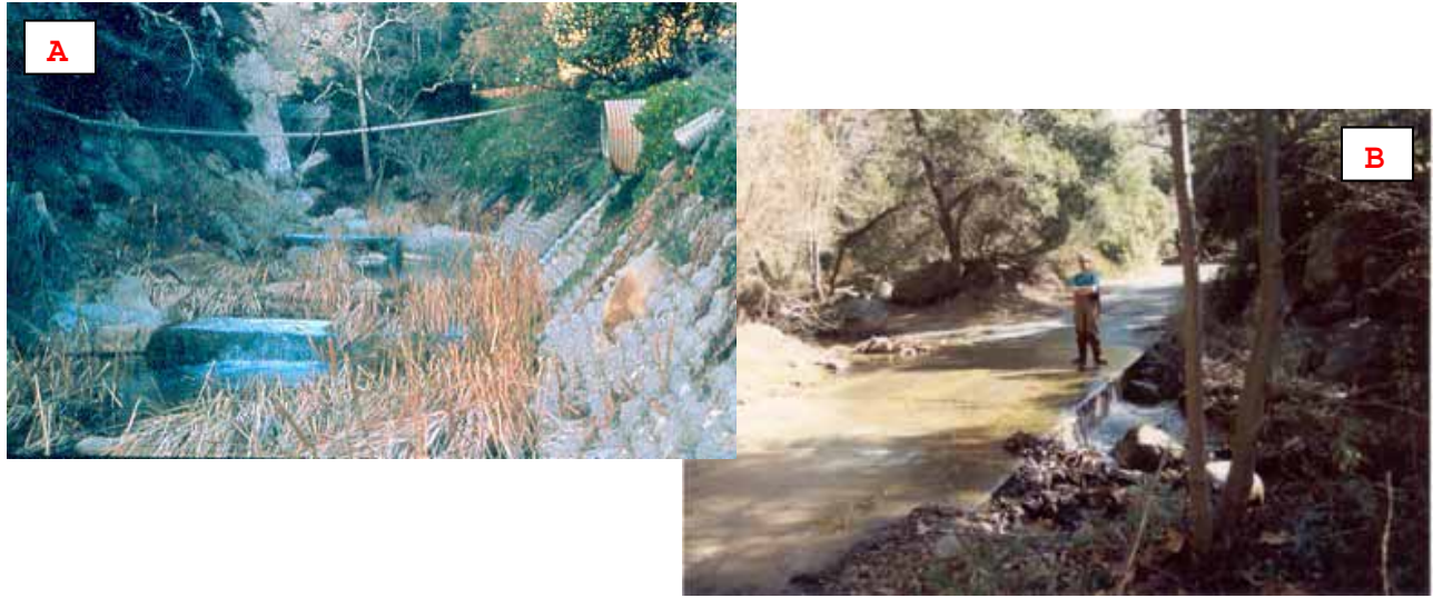
Figure 6. Southern California stream urbanization: Concrete channelization (A) and Ford crossing migration barriers (B).
