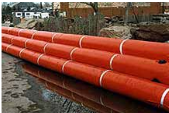
Figure 29. Example of bladders for temporary weir.
