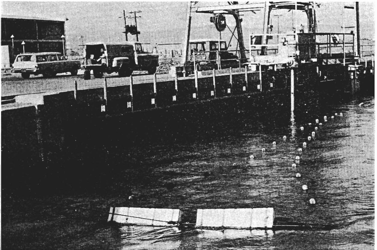
Figure 5. Fyke net in canal just upstream from primary louvers. Net is being pulled ashore by cable attached to net-pulling bridle.
