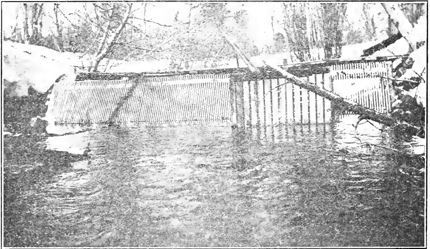
FIG. 14. Racks and trap on Taylor Creek, Lake Tahoe, April 1, 1922. Such temporary racks are utilized in securing black-spotted trout for spawning purposes.
