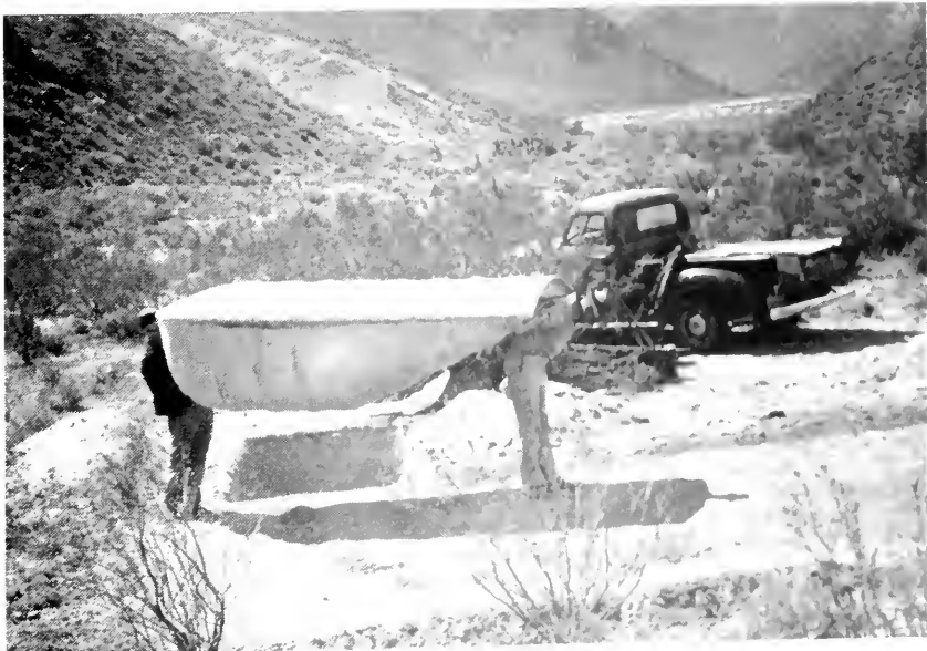
FIGURE 4. Installing one of the new pipe-pipe water troughs.
