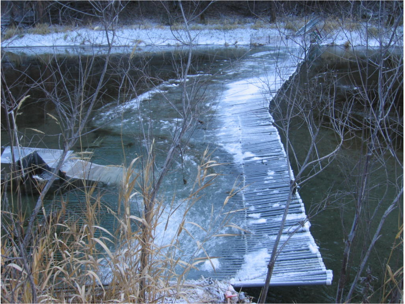
Figure 2. Scott River Fish Counting Facility located in Siskiyou County, California 2010.
