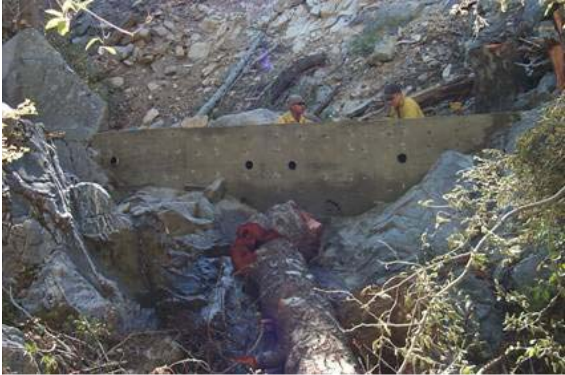
Figure 3a. Enhanced fish barrier at Little Rock Creek. (photo by Bill Brown, USFS)
