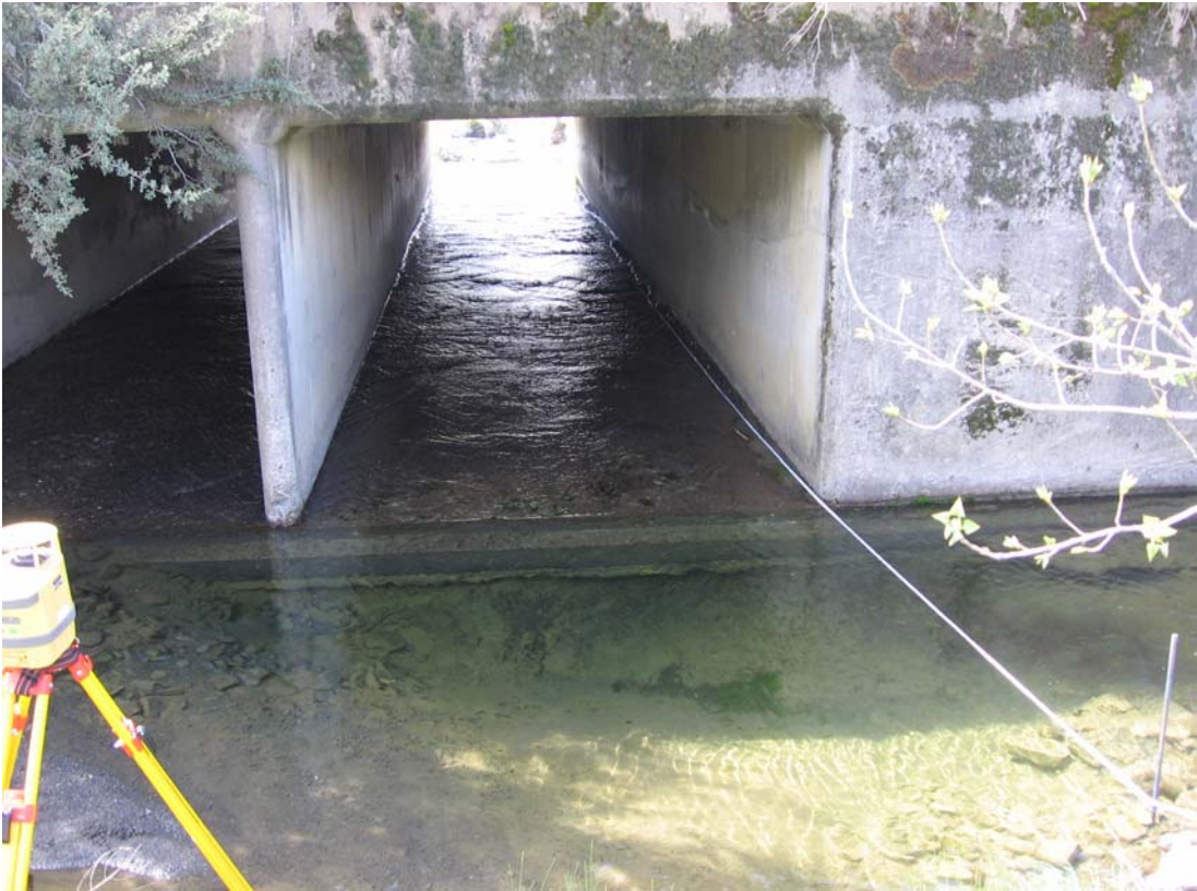
Site # 6- Unnamed Tributary to Dry Creek/PM 9.98; Hwy 36 W Teh.
