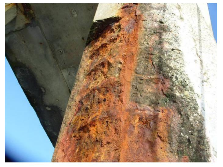
• Exposed corroding reinforcing steel on pile
