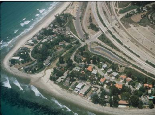
Rincon Creek Estuary (Courtesy California Coastal Commission)
