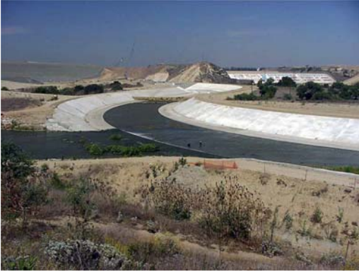
New and Old Prado Dams – Santa Ana River
