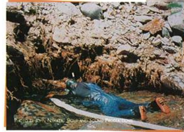
Dredging the streambank has exposed plant roots and washed silt into the stream. It has also destabilized the bank, which leads to further erosion.
