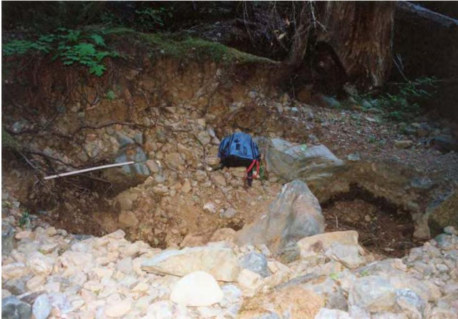
Figure 3. During summer 2001, an estimated 7 cubic yards of soil was excavated from 20 ft of streambank (bottom photo) and 5 cubic yards placed directly into Briggs Creek (top photo).
