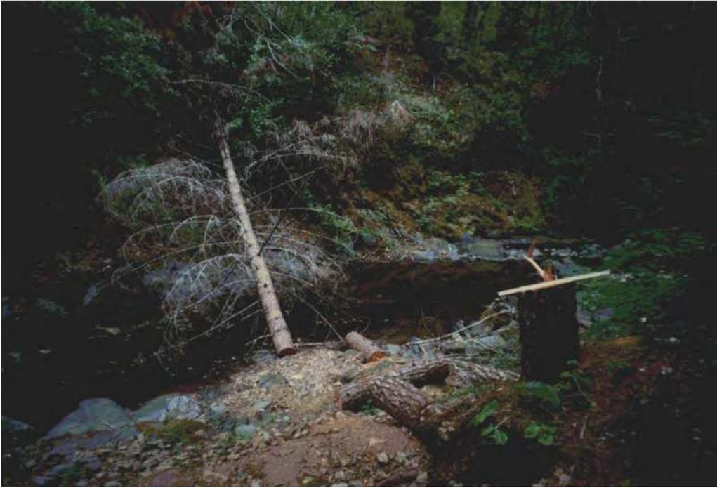
Figure 11. During summer 2001, a live 14-inch diameter Douglas-fir tree was felled into Briggs Creek and bucked. Streambank below fallen tree was excavated.
