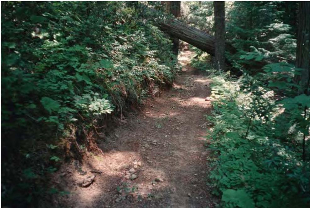
Figure 10. During summer 2000, a hiking trail along Left Fork Sucker Creek was widened by excavating soil from hillslope to accommodate all-terrain-vehicles (ATVs) used by miners.
