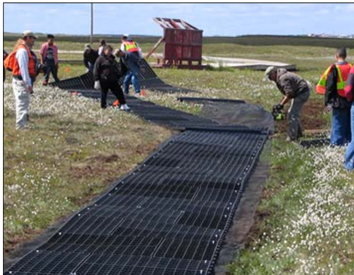
Installation of GeoBlock trail hardening panels in Pinkey's Park last summer in Bethel.
