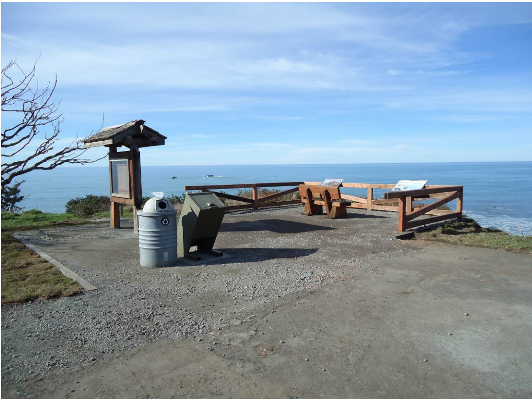
Photo 8. After the installation of the trail head.
