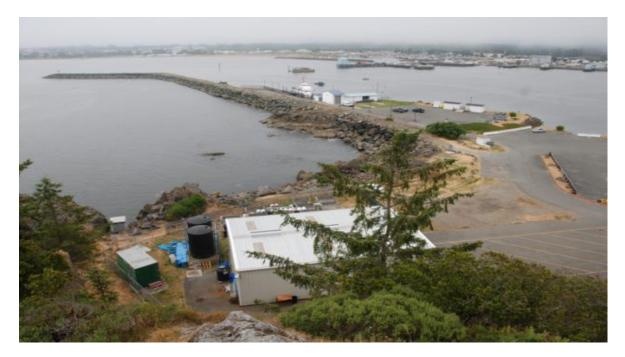
Figure 5b. Photograph taken from Whaler Island looking north/northeast into Crescent City Harbor. Note the Coast Guard duty station. The storage building in the bottom center of the picture occurs at the base of the cliffs that were created from mining the island to create the breakwaters.
