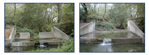
However, in all the years that the flashboard dam was in place, the restriction of the high water flows caused bed-load to settle upstream and it formed a stable gradient of the stream. When the inner walls were removed, it allowed the water to flow much faster, and the stored sediment upstream was washed through the structure. The channel bed head cut traveled upstream approximately 200 feet and perched a culvert that was installed at the prior bed elevation.
