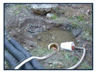
10. Sometimes during construction, the water diversion may be accidentally damaged. When this happens, the diversion needs to be sealed quickly before the water from the pipes overwhelms the pump at the downstream end. With some advanced planning, this can be done quickly.
