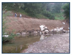
The project plan was to stabilize the toe of the bank and slope the upper banks so they would support vegetation as the primary stabilizing measure. Rock toe protection was chosen to ensure that the bank did not undercut further and threaten the sewer line.
