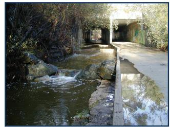
Rock weirs were constructed in the natural channel downstream from the culvert and adjacent to the longer concrete apron. The boulders were anchored into the natural bank on one side, but we were not able to key rocks into the concrete. Instead, the boulders were placed up against the concrete and attached by cables. Each weir dropped and had a narrow spillway for fish passage. By all appearances, the structures should have worked fine.
