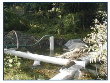
flow out of the work site. An excavator was used to dig a hole approximately 7 feet deep. In the hole was placed an 8 inch PVC pipe with slots cut in it to let water flow into the pipe. The channel bed was refilled with the pipe embedded in the channel bed. A submersible pump was placed into the pipe to pump the water down.
