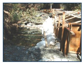
slurry and contaminated pool water. We found that if we pumped the slurry out too fast, we would pull the groundwater away from the pool, and the fish began gulping for air on the surface. We shut down the pump and the fish were fine. We adapted to running an electric pump for short periods and then turning it off. This was sufficient to manipulate water pressure and keep slurry water from entering the pools, and it kept the fish oxygenated and the water clean.
