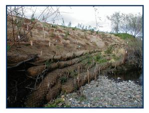
maintaining high soil moisture and suppressing most grasses and weeds. It also prevents raindrops or irrigation water from hitting the soil below and helps prevent washout of soil under the netting. Together, the netting and mulch help the native plants thrive while substantially reducing maintenance effort and cost.
