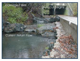
weirs, footer rocks were installed, and these made for strong resistance once flows had mobilized enough bedload to expose them. Under these conditions, the main channel resisted flow better than the substrate under the road. So, flanking doesn't just happen on the surface.
