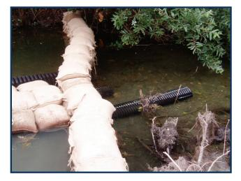
In most cases, these dams are constructed with sandbags filled with washed sand, rather than gravel, and without plastic sheeting. Straw bales may also work to block flow and filter sediment. In most cases, these weirs are not sealed because pumps will move the turbid water
