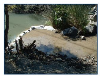
pumps. Pumps pull turbid water from the work zone and deposit it outside the stream channel, usually into a sediment basin or onto adjacent land where it won't run back into the stream.
