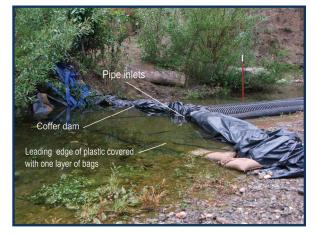
materials because as the dam impounds water, the volume and elevation of water upstream builds up and can flow around a coffer dam that is too small.
