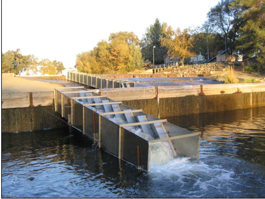
Figure 1. Bellota Weir's staggered fish ladders.
