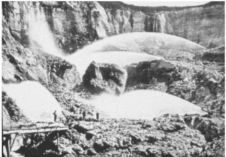
Giant water cannons, or monitors, were used at Malakoff Diggins to erode gold-rich gravels from 300- to 500-foot high cliffs. Gold was separated nearby and resulting tens of millions of tons of sediments were released to local streams and rivers (circa 1860).
