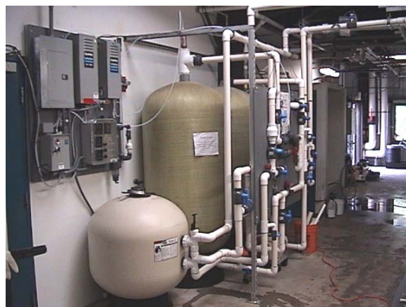
Figure 13. Ozone system used to treat make-up water to all recirculation systems.
