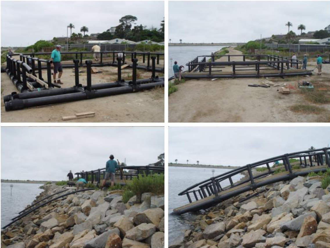
Figure 6. Construction and launching of Agua Hedionda Lagoon growout facility. Note flexibility in HDPE pipe.
