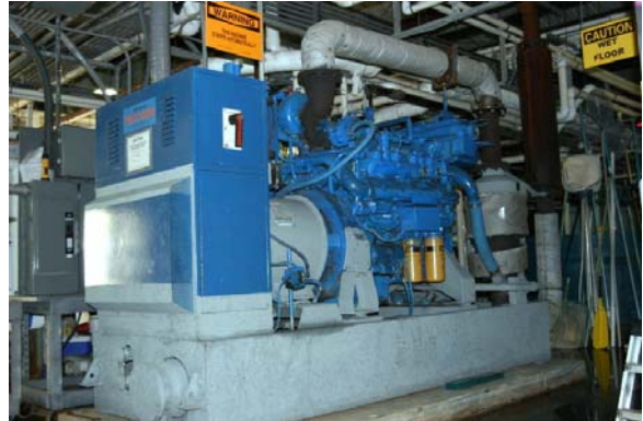
Figure 9. 225KVA emergency generator inside hatchery building
