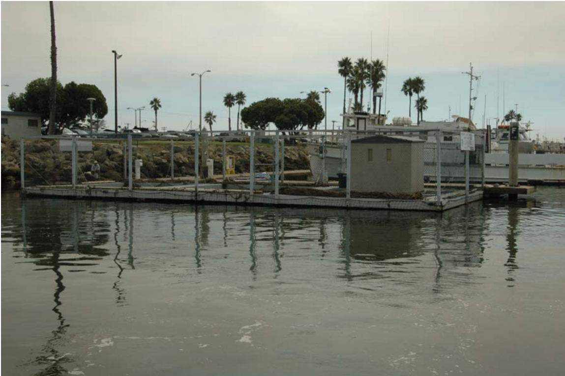
Figure 25. Channel Islands Harbor white seabass delayed release netpens. The copper treated netpen encloses a volume of 116 m 3 . One thousand two hundred nineteen kg of juvenile white seabass were released from the facility on September 15, 2005.
