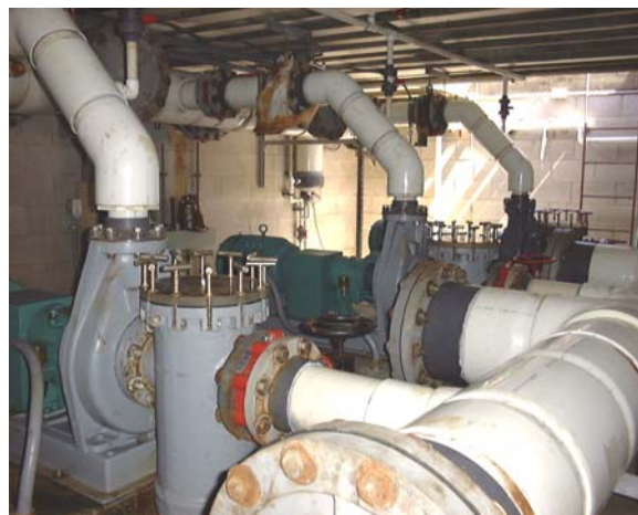
Figure 11. Primary seawater pumps housed in an insulated vault for noise dampening.
