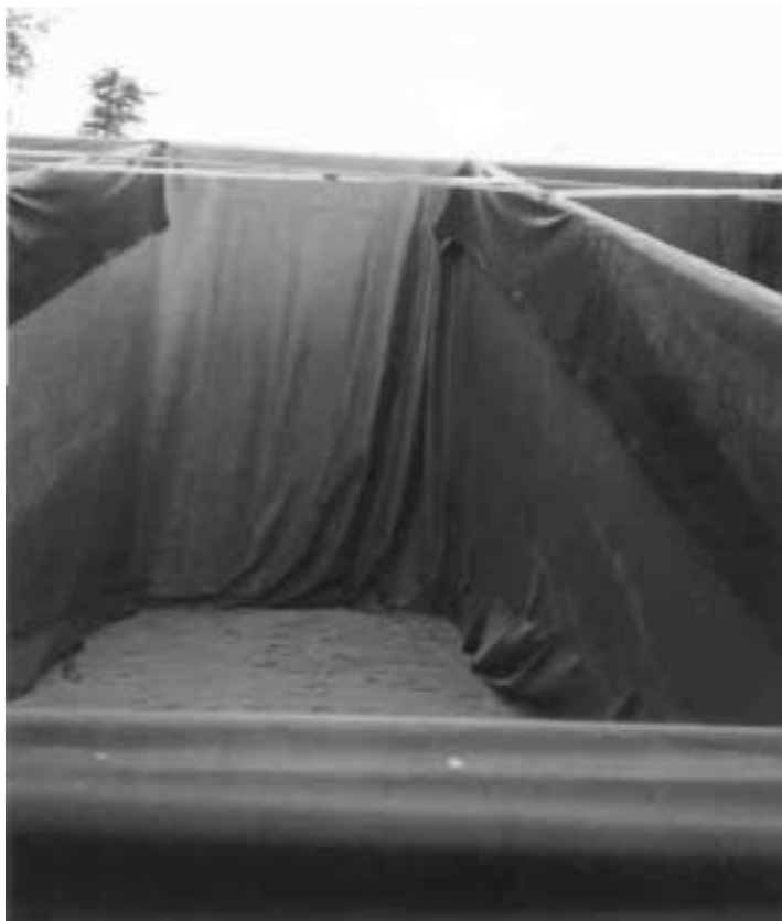
Figure 7. View of a Cell filled with Wasterock
