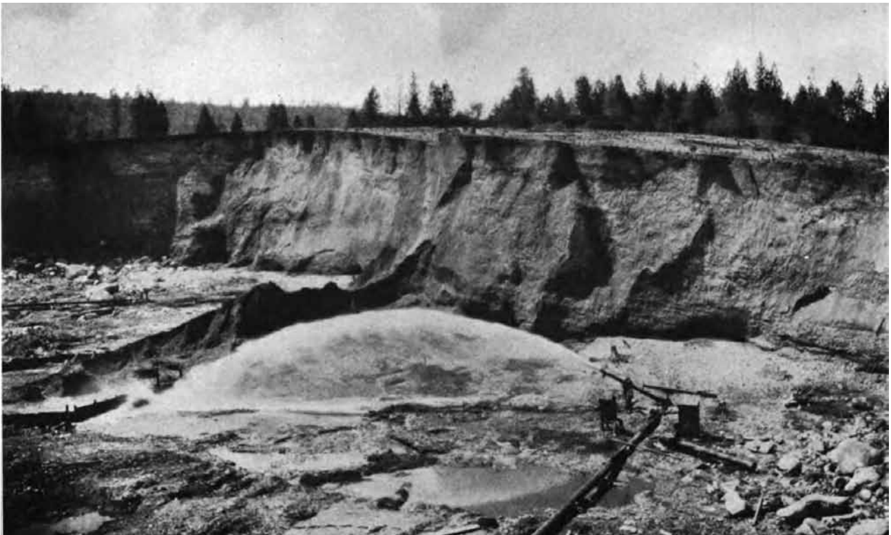
Figure 1.13. Hydraulic mining. The caption of this photograph, which is shown as Plate I of Grove Karl Gilbert’s treatise on hydraulic mining debris (1917), reads: “A hydraulic gold mine. The water is conveyed by pipe, under a head of several hundred feet, and delivered through a nozzle that can be turned in any direction. The jet washes the auriferous earth from the cliff and thence to a sluice, seen at the left. The sluice is several hundred feet long and contains pockets of mercury by which the gold is caught. (photo by Gilbert 1908, from Gilbert 1917)
