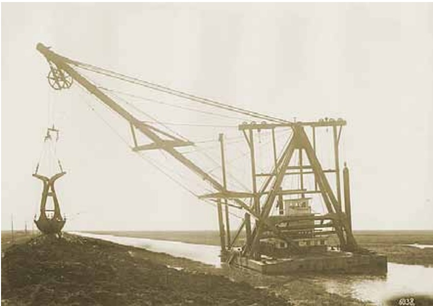
Figure 1.15. Clam-shell dredge building levees. The clam-shell dredge, Vulcan, is shown building the height of an artificial levee along an unknown waterway. After initial reclamation efforts, where levees were built primarily by Chinese laborers, dredges were used to build higher levees to keep out the tides and floods. (McCurry Foto Co. ca. 1910, courtesy of the California History Room, California Sate Library, Sacramento)
