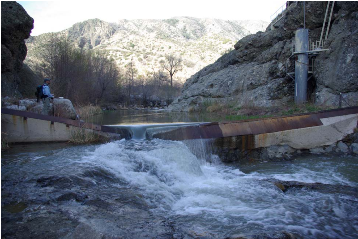
Figure 3. Photograph of USGS gaging station near confluence of Piru and Buck creeks
