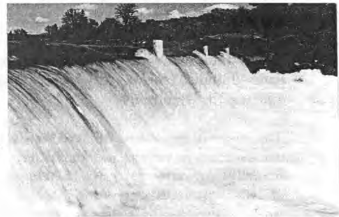
FIGURE 8. Fish barrier, a 110 x 6 ft structure with a concrete apron, located above Lake Britton.
