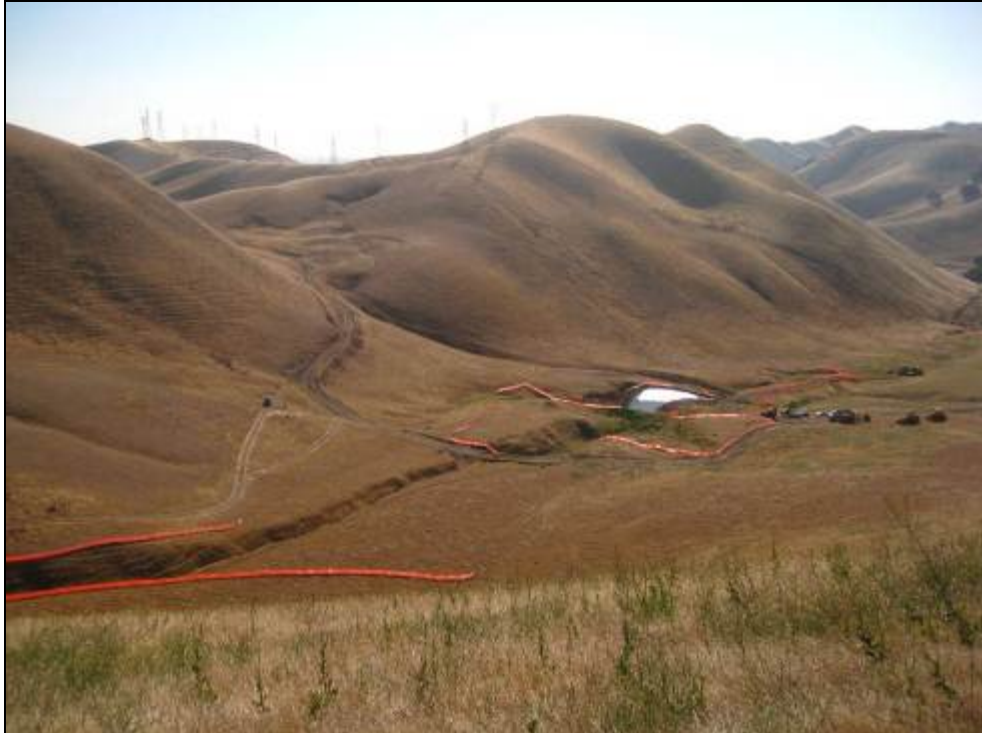
Figure B-1. Silt / Wildlife Exclusion Fence installation. (4 August 2011)
