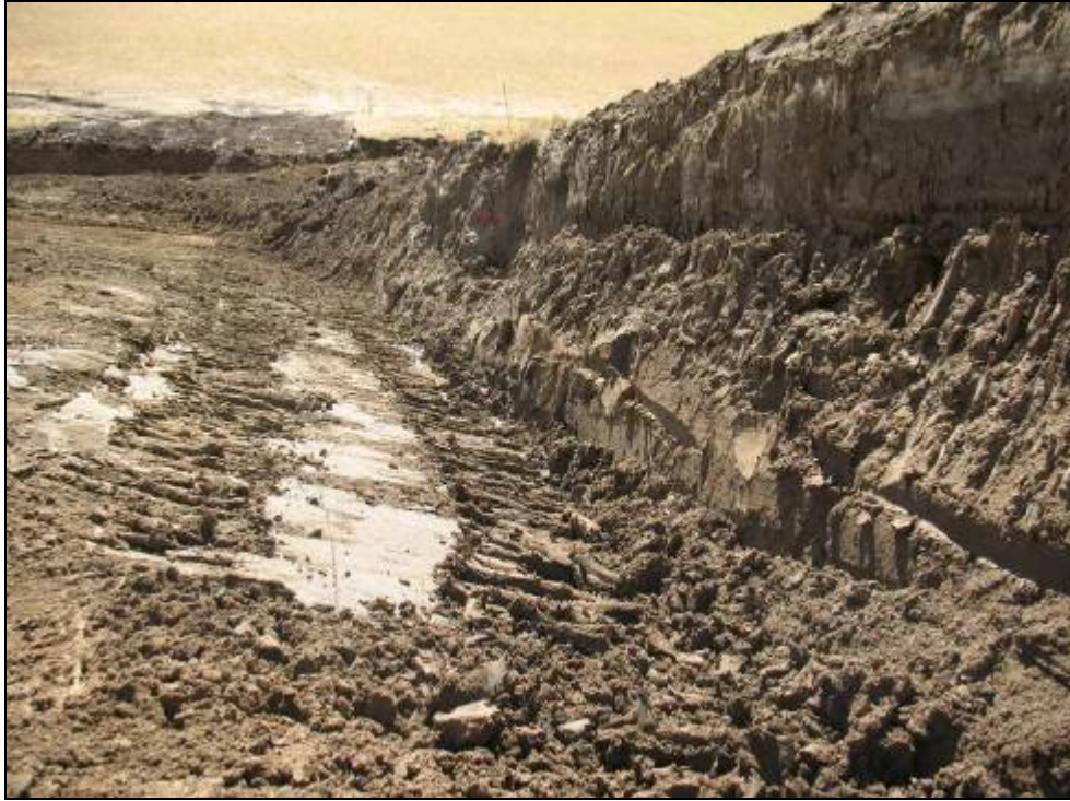
Figure B-3. Alluvial Valley sub-grade excavation at the upstream transition area. (15 August 2011)
