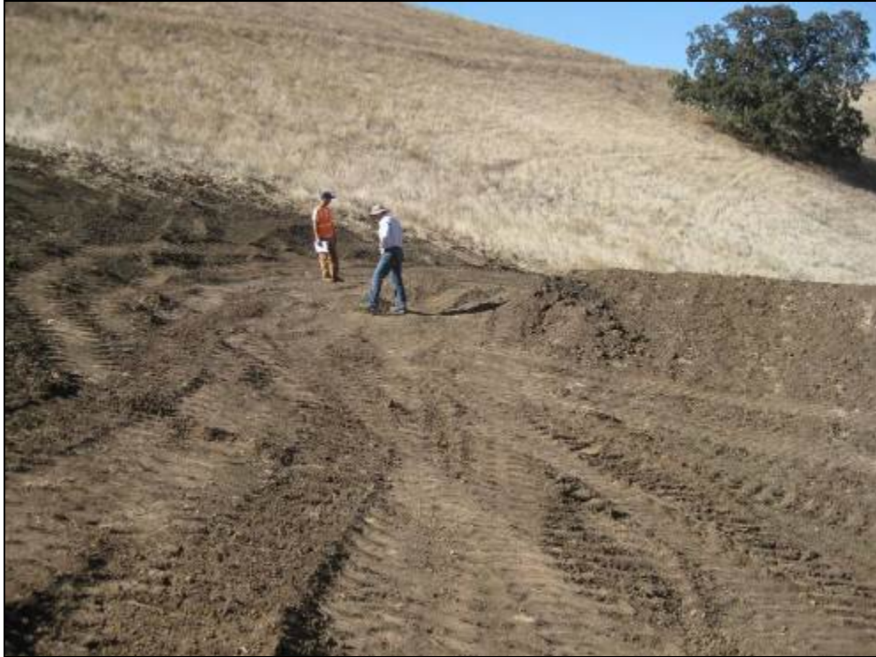
Figure B-7. Rough grading at the CTS Pond. (18 October 2011)
