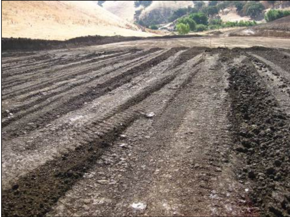
Figure B-5. Imported clay placement in the Alluvial Valley. (18 August 2011)
