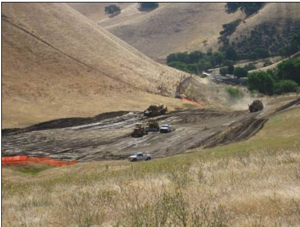
Figure B-2. Alluvial Valley sub-grade excavation. (9 August 2011)
