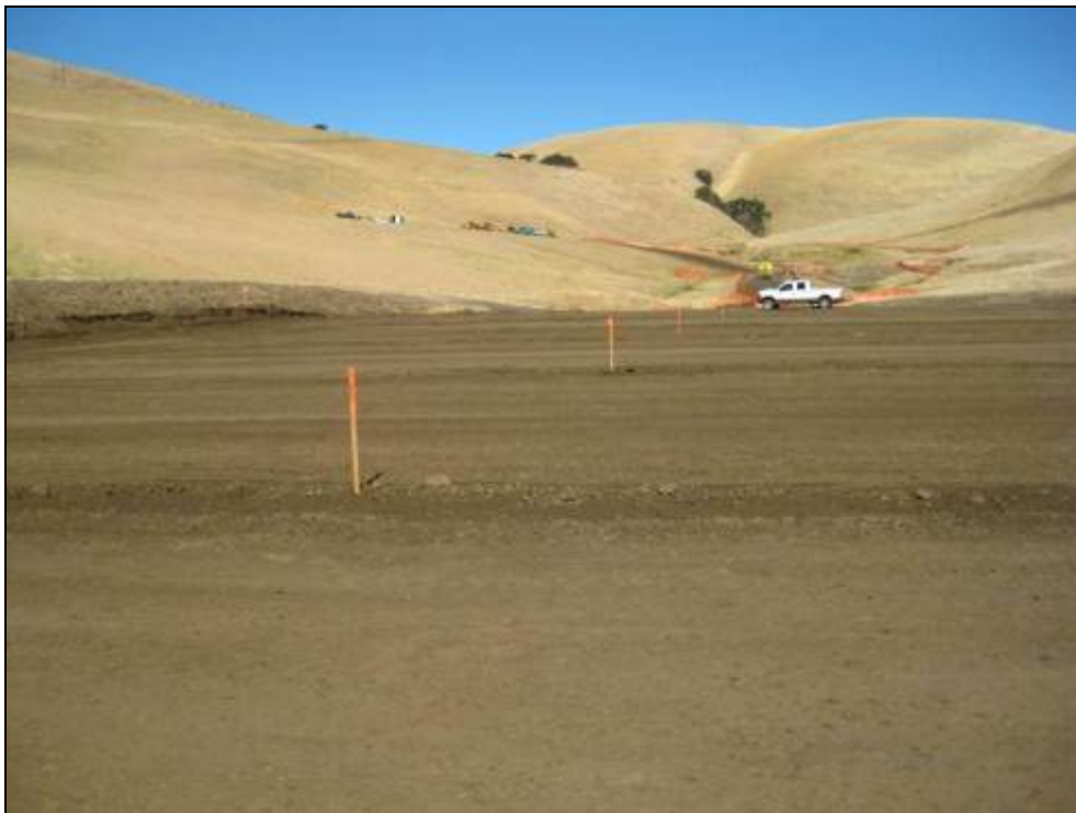
Figure B-6. Soil placement between the clay risers at the Alluvial Valley. (6 September 2011)
