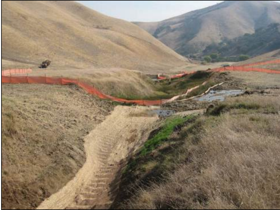
Figure A-9. The Channel Restoration Area following seeding and straw placement. (9 November 2011)
