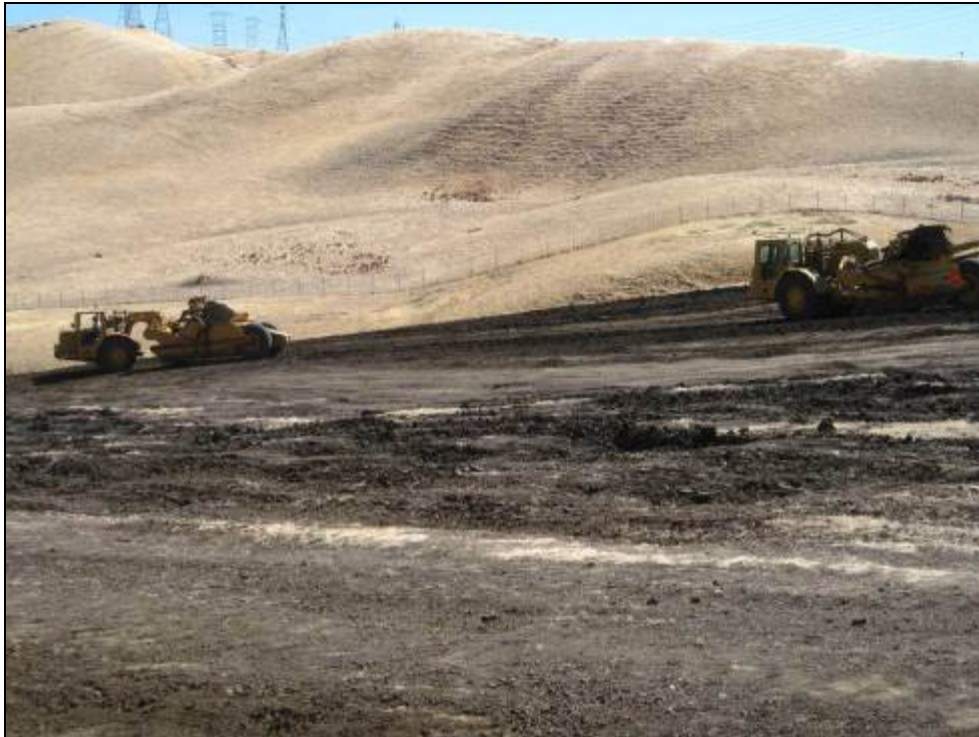
Figure B-4. Soil harvest from the Clay Borrow Area. (18 August 2011)
