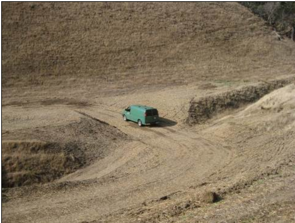
Figure A-10. The new Ranch Road Crossing following seeding and straw placement. (9 November 2011)
