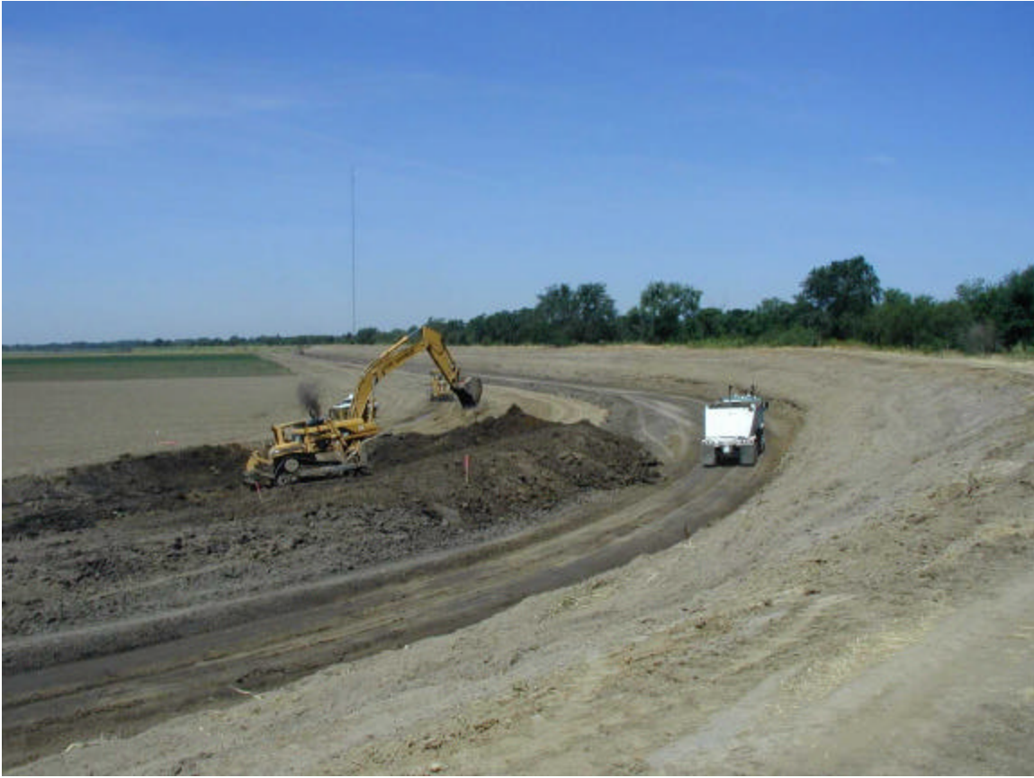
Figure 2 – Resloping of interior face of levee on McCormack Williamson, summer 2001. The surface is at a 5:1 slope.
