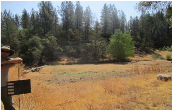
Sediment build-up behind Swasey Dam.
