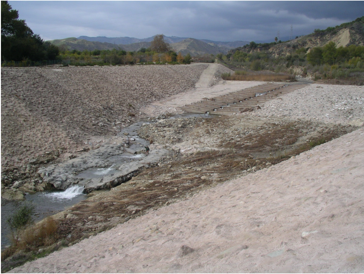
Grade control and fishway before 2005 failure
