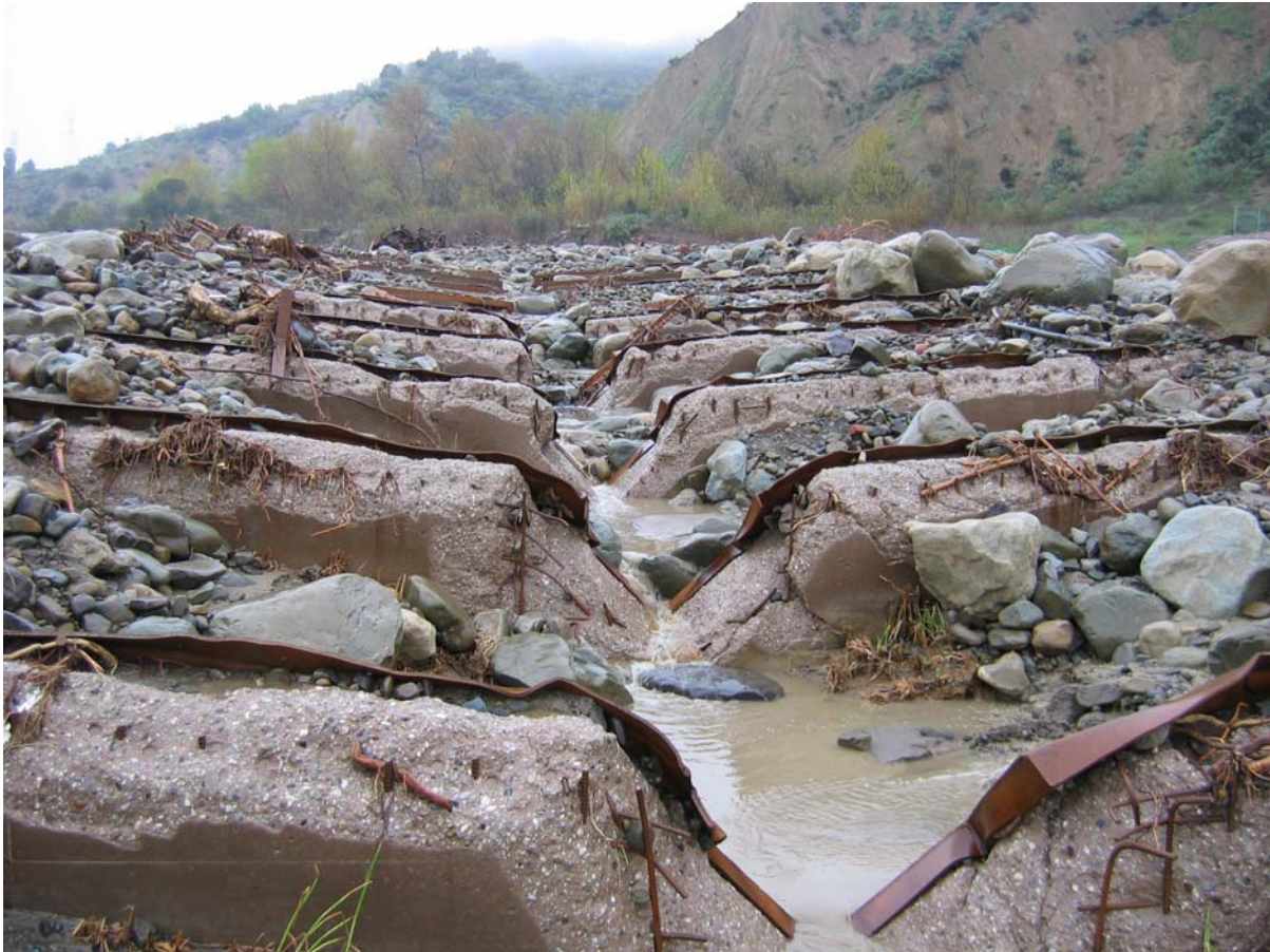
Fishway failure following January 2005 flows
