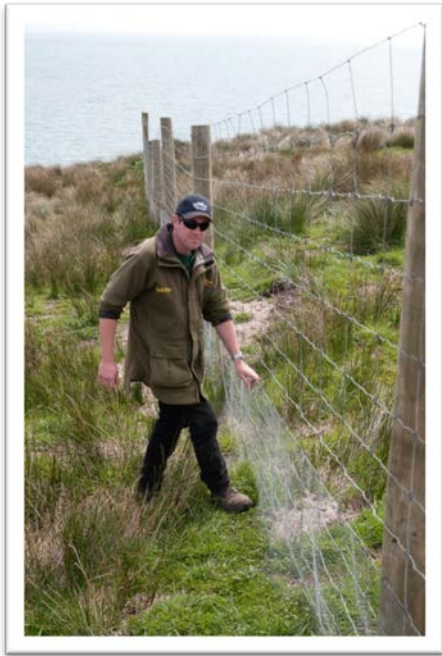
Photo 2. Martin showing me the fine mesh base complete with 'footing'. Note how the plants are binding into this and apparently helping to keep it pegged down and deter rabbits digging through. The height of the fine mesh is about 500mm - high enough to stop bunnies jumping through. (photo: Jaime Newman)
